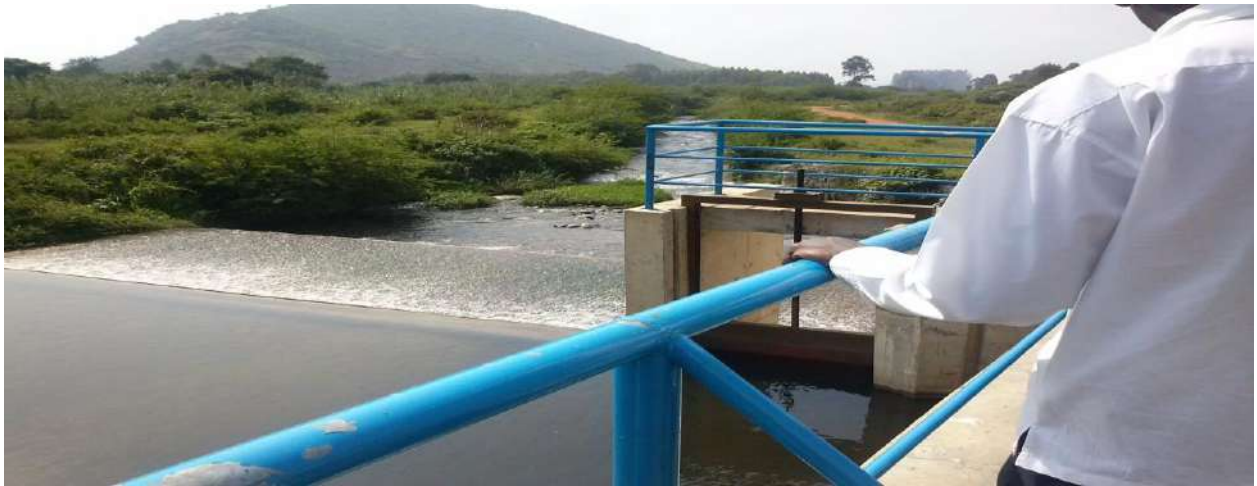
Figure 3.4: One of the renovated Water reservoir facilities at Mobuku irrigation scheme
