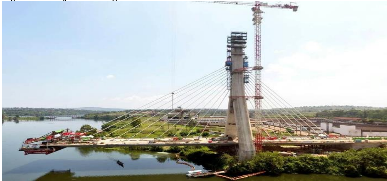
Figure 4.4: Jinja Nile bridge under construction
